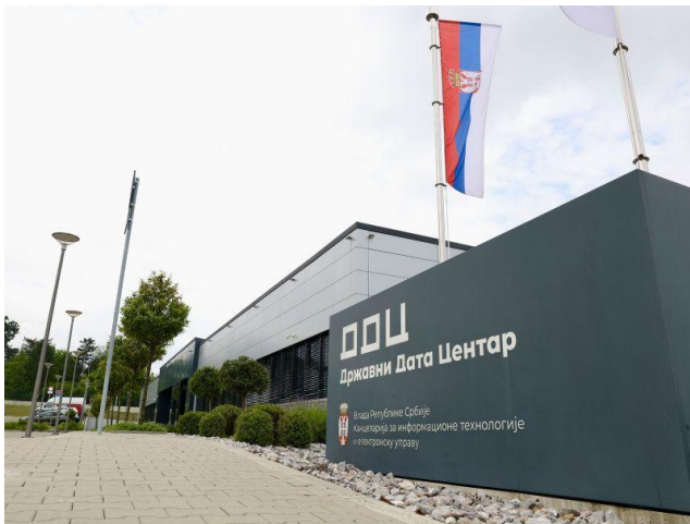
Government Data Center
