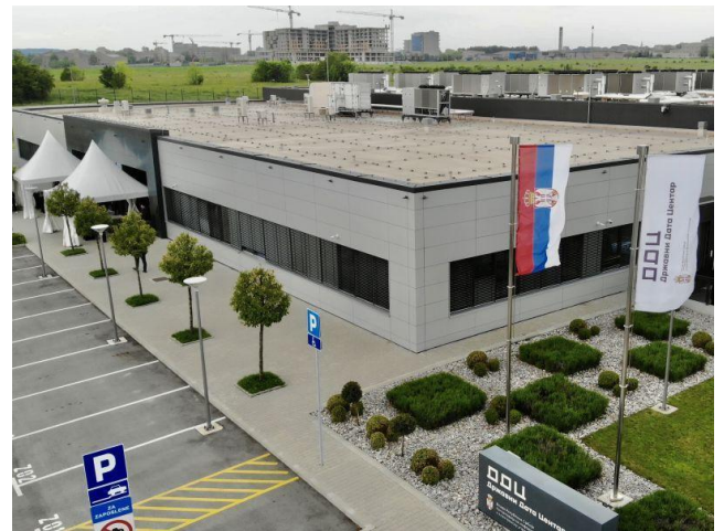
Government Data Center
